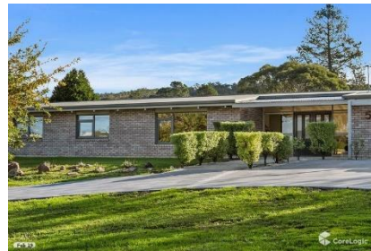
5 Hopfields Road, Margate, Tas 4 bed, 2 car, 2 bath house $720,000 Knight Frank Tasmania
